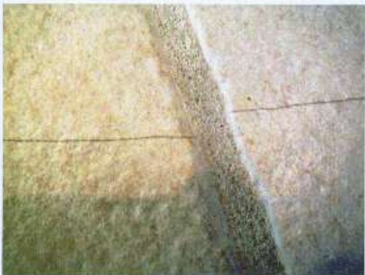
1/14/2009 Cracked floor tiles
