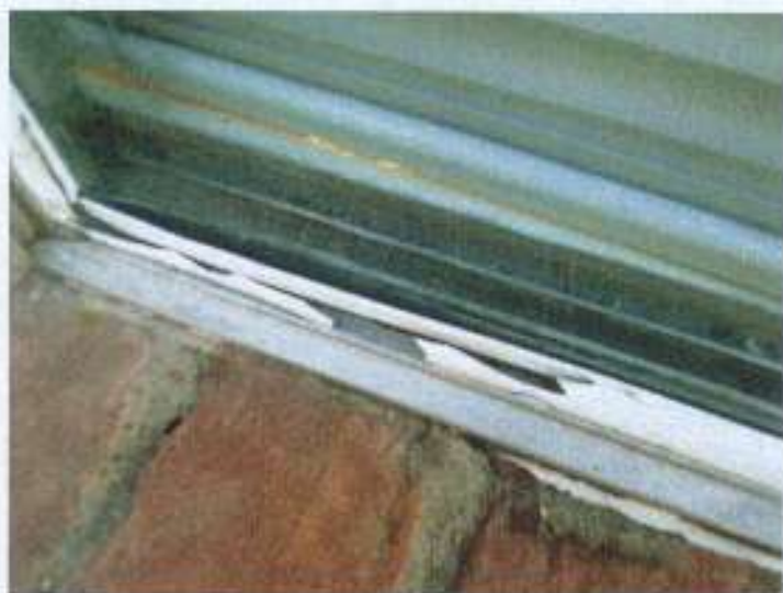
1/14/2009 Decayed plastic window pane strips
