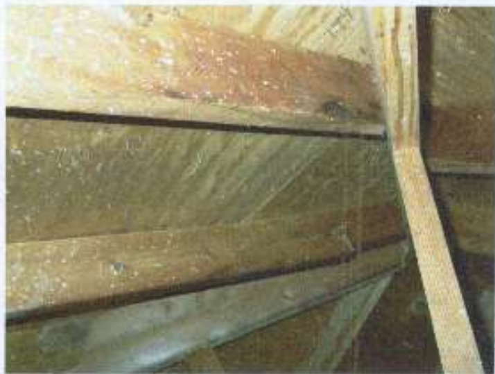
1/14/2009 Cracked rafter in front attic
