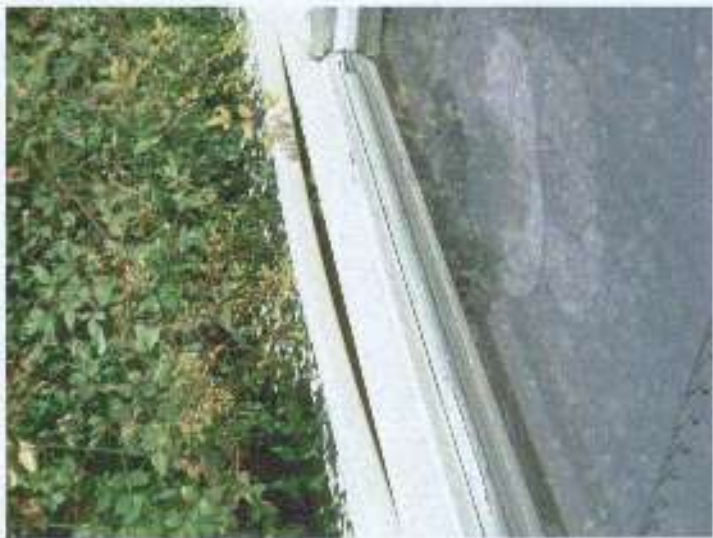
1/14/2009 Loose vinyl siding at back of breakfast room
