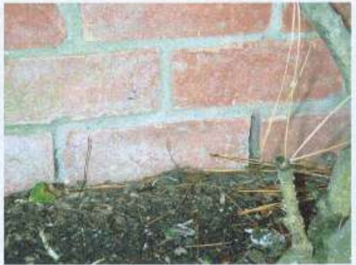
1/14/2009 Soil above slab in spots
