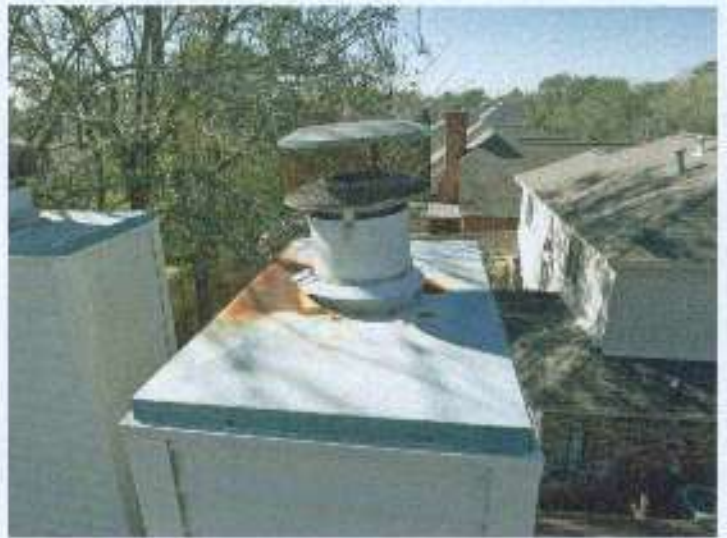
1/14/2009 Rust on chimney cap
